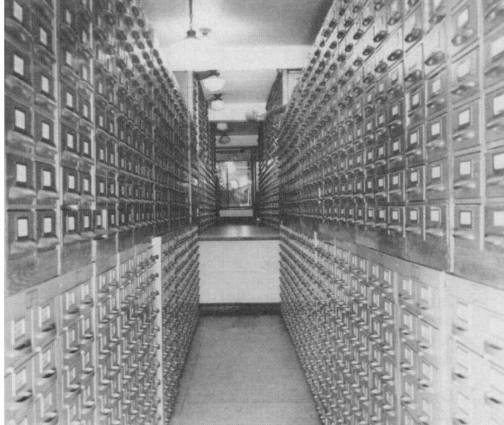
Figure 3-16: IBM-705 computer recorded most of the climatological data on over 300 million punch cards filed in these and other drawers at AWS Data Control Division.
