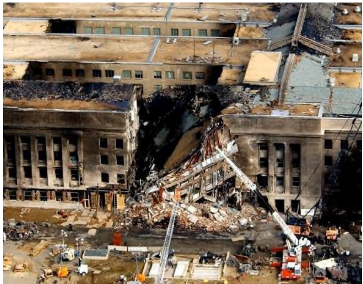
Figure 8-6: Pentagon damage from 11 Sep 2001 Terrorist Attack
