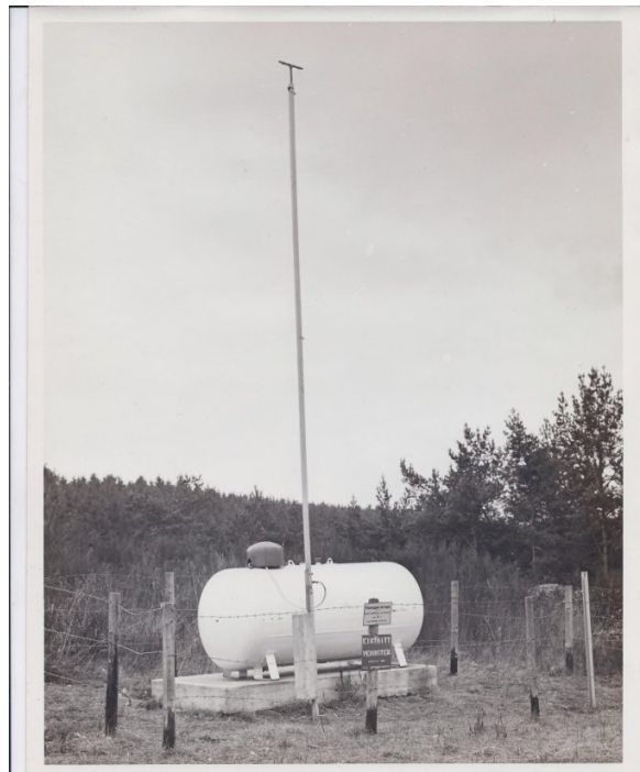
Figure 5-17: Manually activated CFDS at Hahn AB, Germany.
