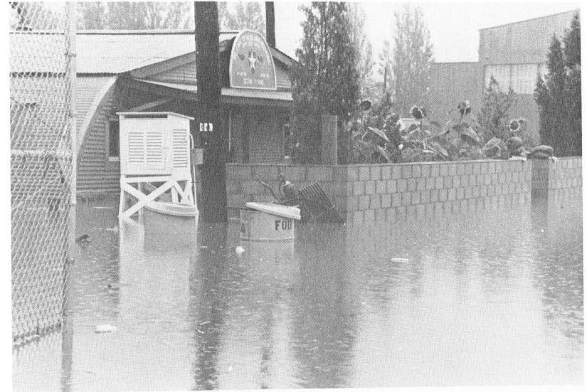
Flooded Operations building at Camp Casey, Korea, in September 1984.
