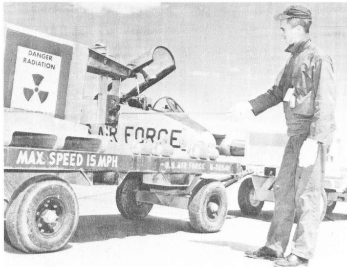
A cloud sample, just removed from a B-57 Martin Canberra and inserted in shipping "pig", is monitored by AFC Thomas O. Summers, 1211th Test Squadron (sampling) in connection with Operation Plumbbob. Other leaden "pigs" on truck are to be loaded. Note the protective gloves and rod used to work the monitor control.
