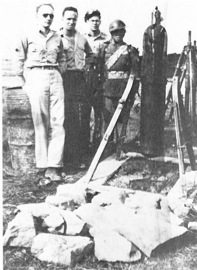
Hydrogen manufacturing Unit, 10th Weather Squadron, Liangshon, China, 1945. Aluminum chips and HCL acid were used to make hydrogen in lieu of helium for upper air balloons. These products were lighter to transport over CBI hump. (L-R: Sgt Elmore Frost, station chief, Sgt Mullins, observer, Lt Brabham, Assist BWO, Chinese Nationalist soldier).
