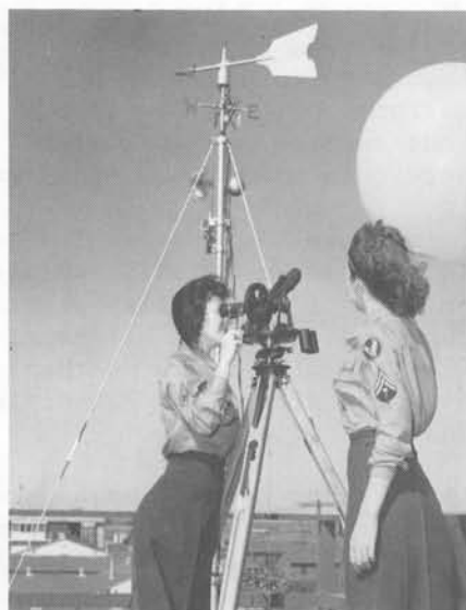
IWS' WAC Cpls Paula Eberstadt (left) and Evelyn Barclay making Pibal run at Minter Fld, Bakersfield, CA, 1944.
