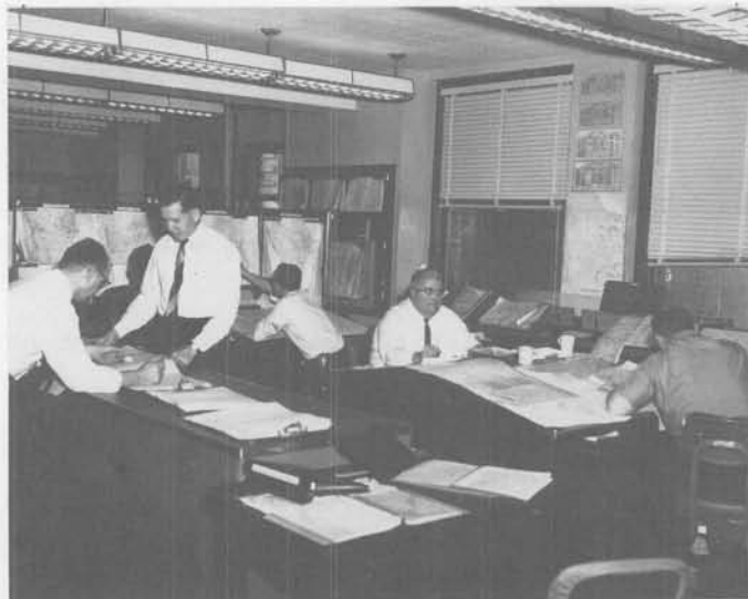
Interior of Kansas City Centralized (Terminal) Forecast Facility showing, left to right in foreground: SMSgt Frank J. Brzeczek, Lt Col James A. Bunce, Lt Col Robert C. Miller, and Maj Neil B. Gardner. In background: CMSgt Claborn I. Gibson and 1/Lt Douglas F. Fenn.
