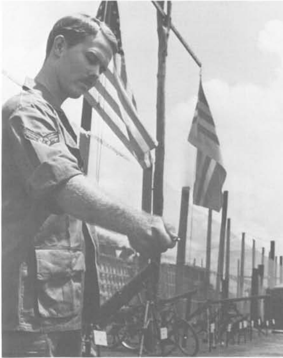
With the 1st Cavalry Division's 2d Brigade at Phuoc Vinh in September 1970, Sgt Ralph T. Wilson, a weather observer with the 5th Weather Squadron's Operating Location B, twirls a sling psychrometer, left, and examines his rain gauge, right. In the background are Viet Cong weapons captured by the brigade.
