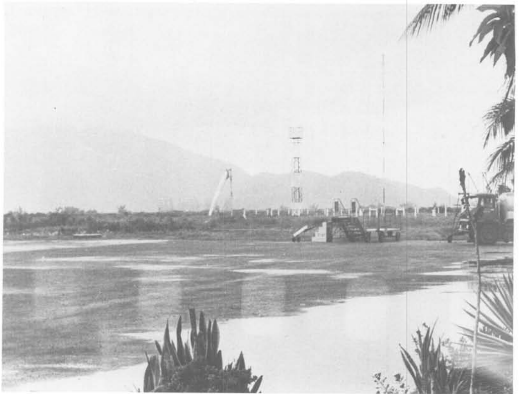
View of Nha Trang airfield with mountain background. Below, Pilot-to-Forecaster Service, base weather station, Nha Trang Airbase, Detachment 20-2, 30th Weather Squadron.
